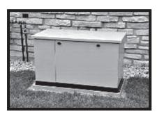
Set the generator onto the pad so that the gravel bed extends several inches beyond the generator on all sides.
